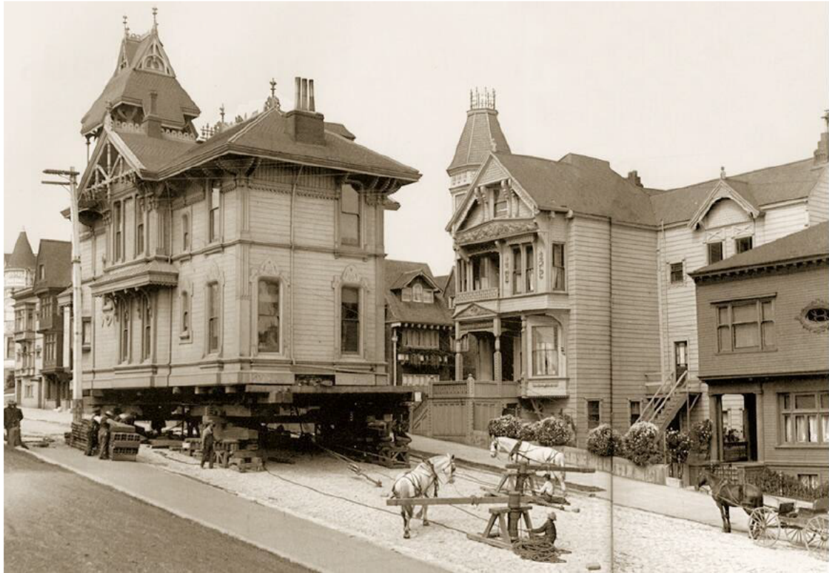
Figure 2: A house being moved by using horses in San Francisco, 1908 (Desroches, 2018)
